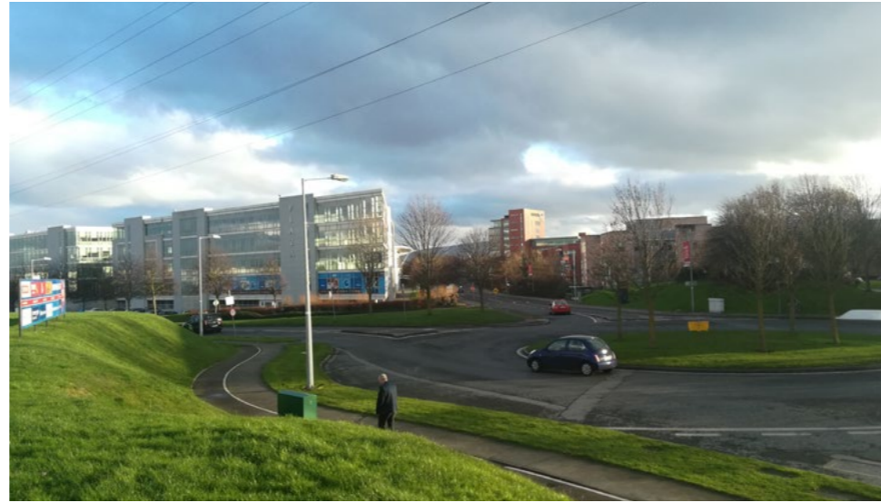
View south, from site to Park West Avenue and Road Intersection
